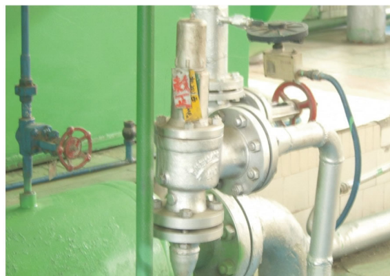
Bellows Safety Valve in Institute of Physics
